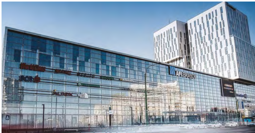
MULTIMODULO Centre commercial AFI BRASOV, ROUMANIE
