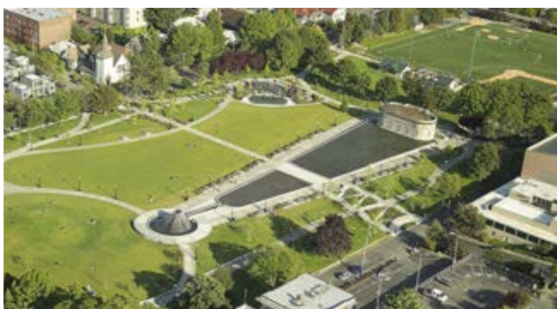
Lincoln Reservoir Cal Anderson Park SEATTLE, USA
